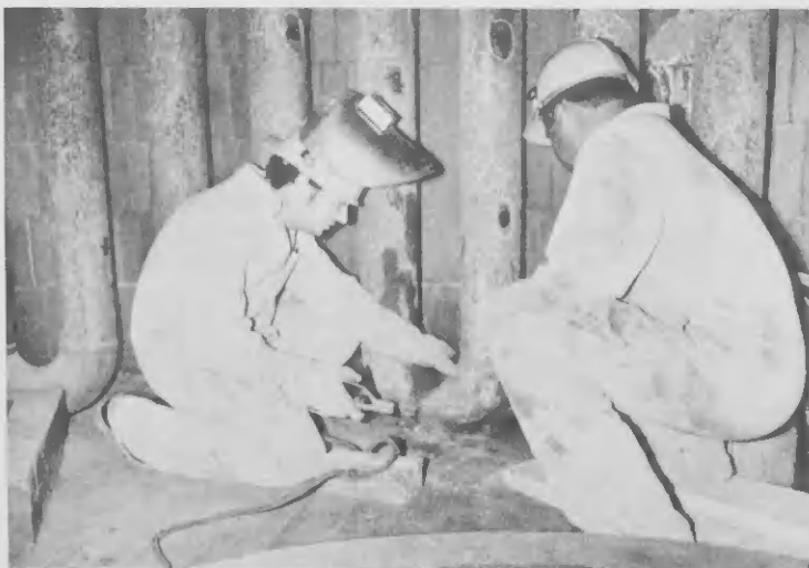
Skilled welders here pause briefly before continuing their task of fitting back the tubes in the KHAR furnace.
